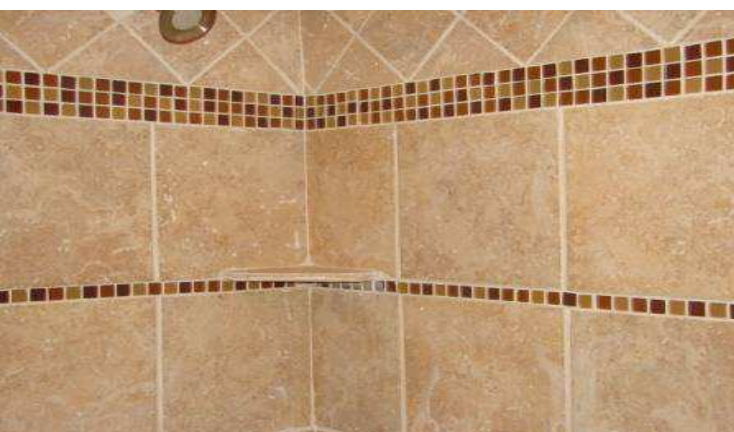
Beautiful Deco Tile and Dedicated Radiant Heat!
