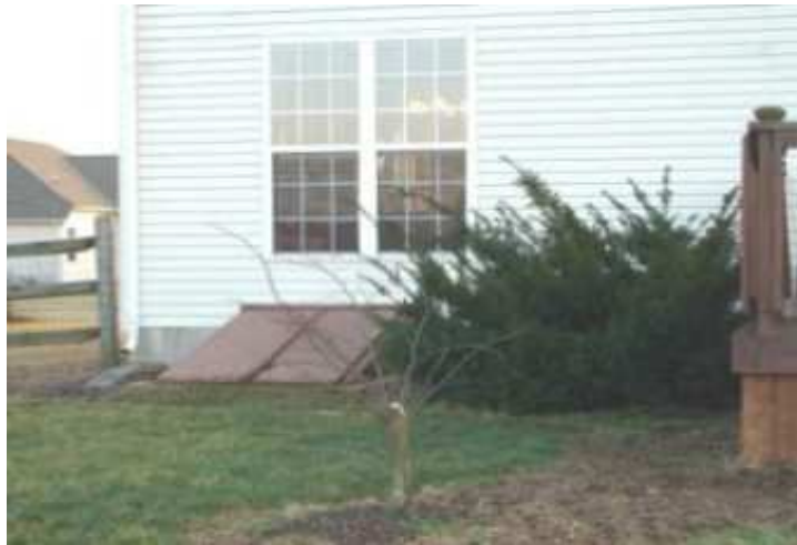
Basement Outside Entry!
